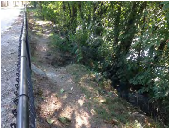
Figure 8 Fence installed to prevent erosion and limit access to steep bank in the Shirlington Dog Park
