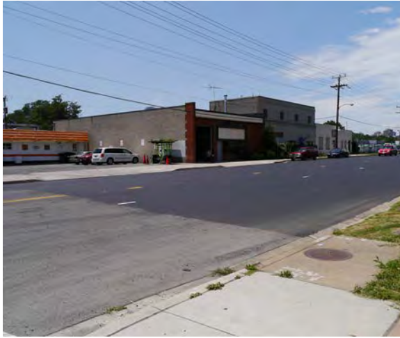
Figure 9 View across South Four Mile Run Drive. The roadway is a major barrier for connectivity between the adjoining neighborhood and the park areas
