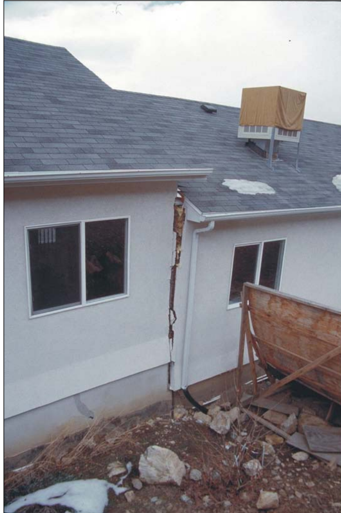
Figure 3. Damage to a house caused by movement of upper part of the Sherwood Hills landslide in Provo. House was condemned in January 2000.
