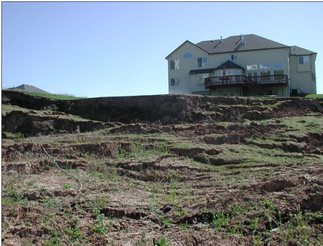
Figure 4. Damage to the rear of a lot caused by movement of the Frontier Drive landslide, Mountain Green in 2001. Losses and stabilization costs of this landslide exceeded $750,000.
