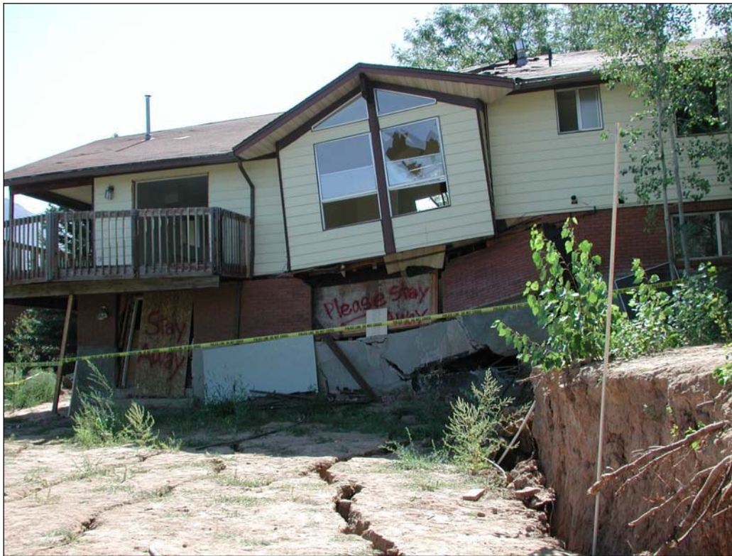
Figure 2. Damage to one of three houses destroyed by movement of the Heather Drive landslide, Layton in 2001.
